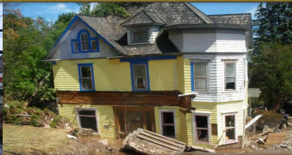
Damage along Schoharie Creek, Prattsville, NY – T.S. Irene, Photo: J. Vielkind / Times Union
