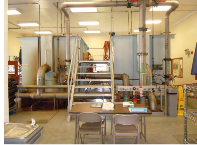
Flooding water infrastructure
